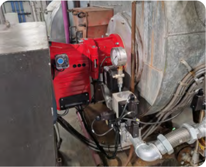
In 2022, this resulted in a change of burners in the five head office boiler rooms
